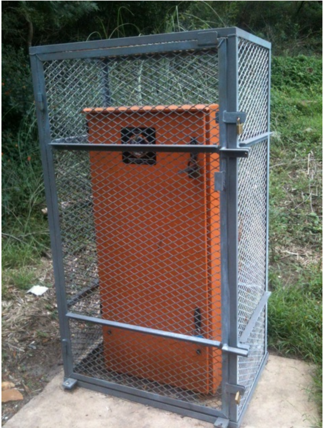
The electric panel to the water pump with secure coverage to keep it save from vandalism.
